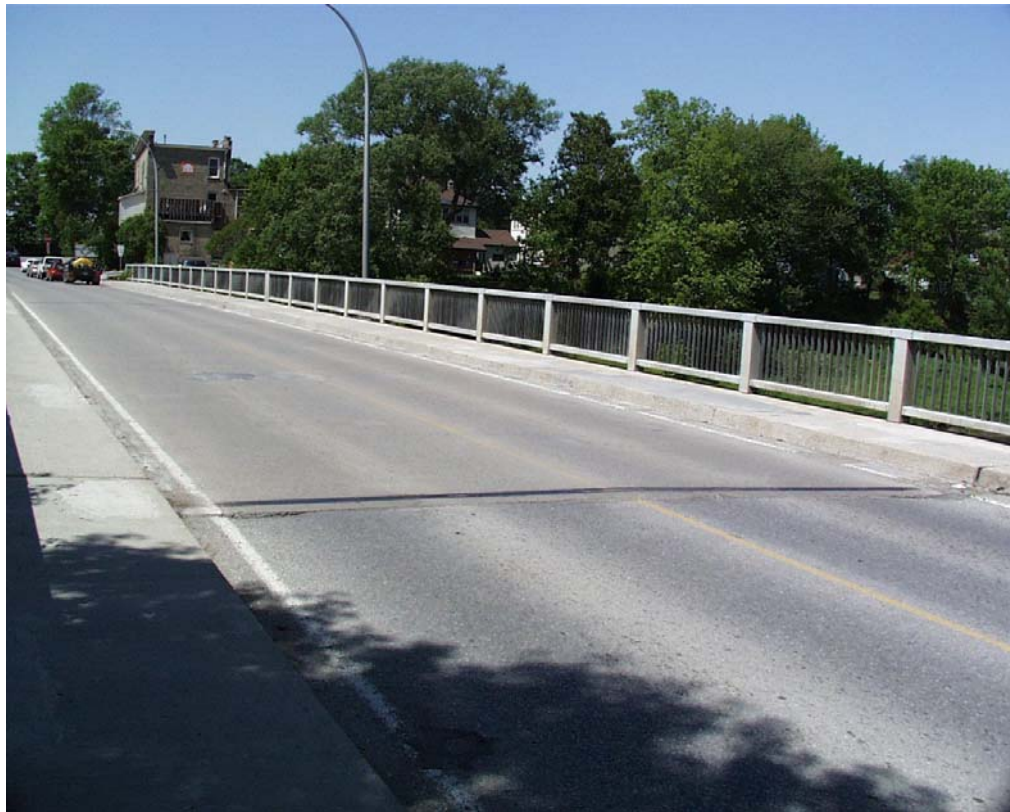
Figure 2 General View Bridge Street Bridge
