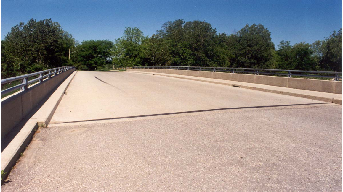
Figure 1 General View Victoria Street Bridge
