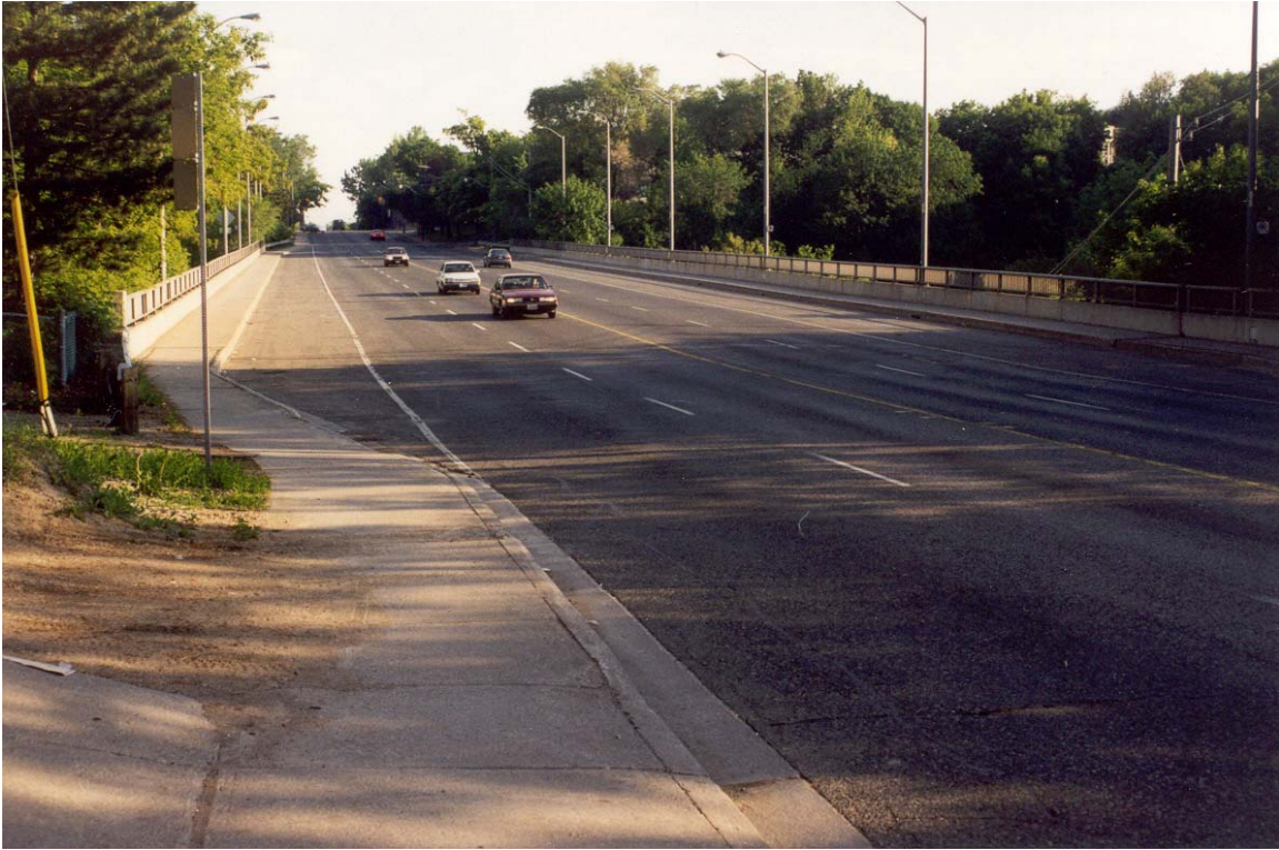
Figure 3 General View Bathurst Street Bridge
